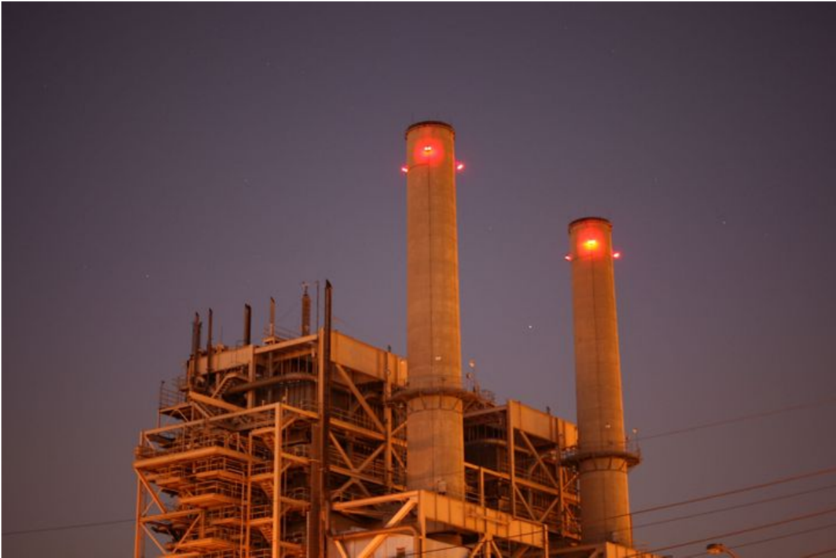
AES Corp.'s gas-fired Alamos Energy Center in Long Beach is one of California's largest power plants. Credit: DAVID MCNEW VIA GETTY IMAGES
